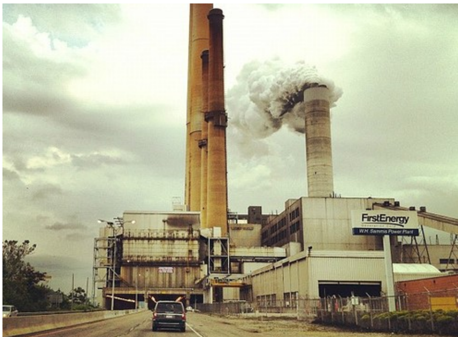
W.H. Sammis plant
